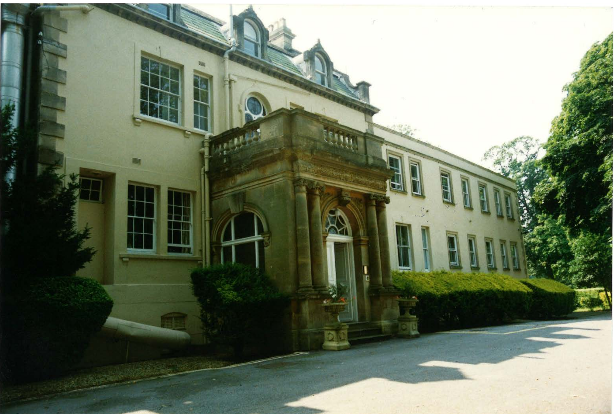
Photo: Mansion south elevation - c. 1990
