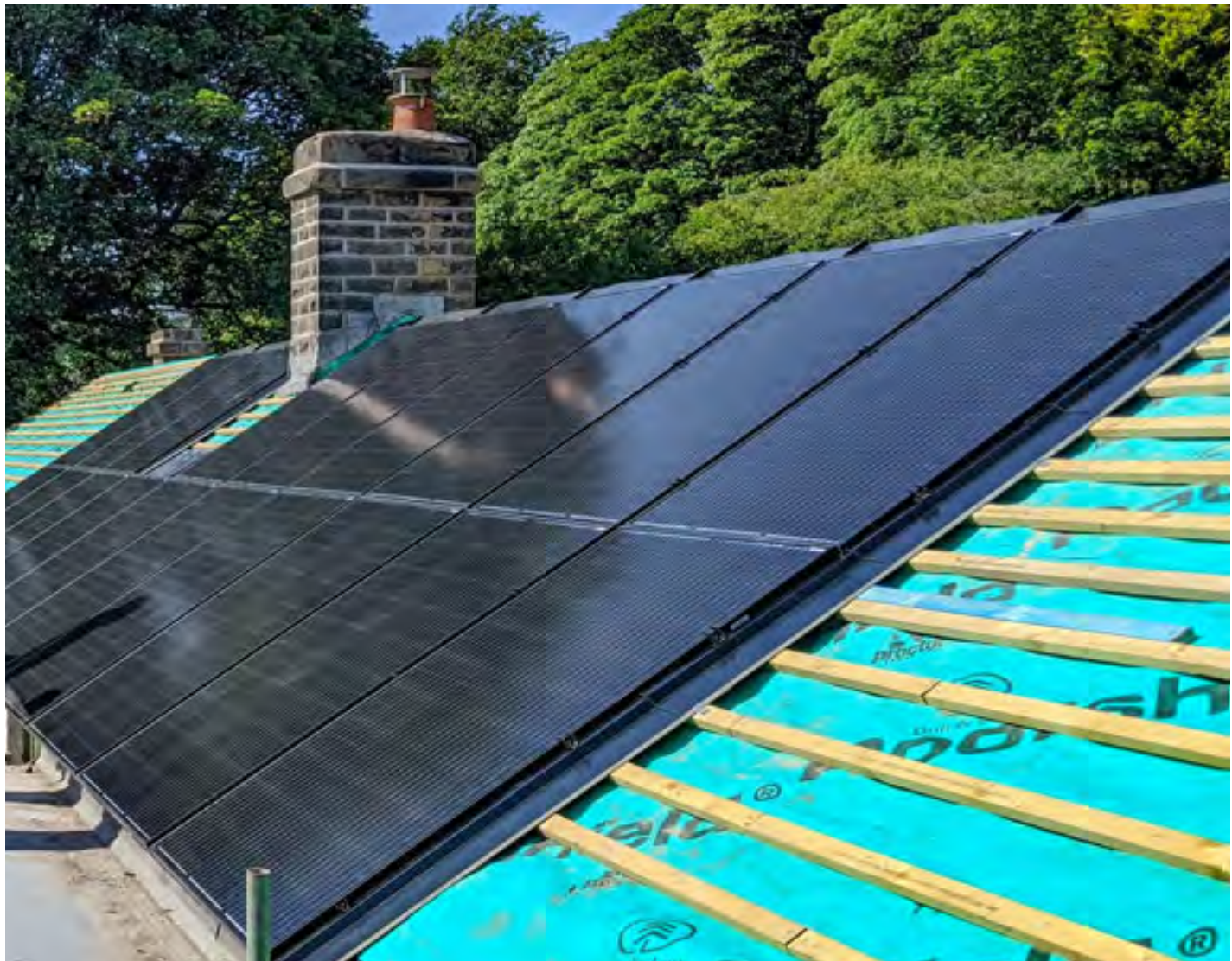
PV array as the roof finish to south
